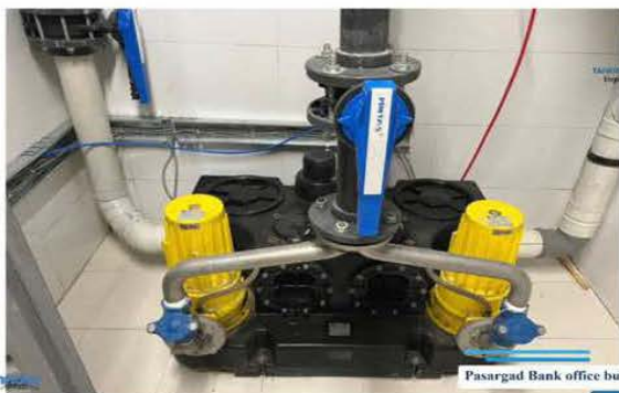
Wastewater lifting pump package
